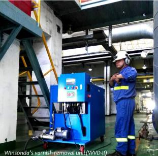
Winsonda's varnish removal unit(WVD-II) was installed at place of compressor reservoir.
